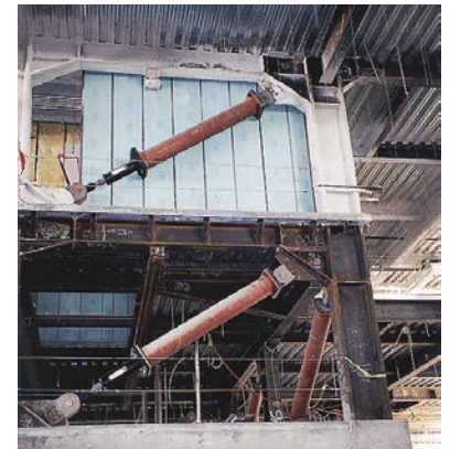
FIGURE 11–17 These huge dampers placed in a building look a lot like huge automobile shock absorbers, and they serve a similar purpose—to reduce the amplitude and the acceleration of movement when the shock of an earthquake hits.
