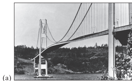
FIGURE 11–20 (a) Large-amplitude oscillations of the Tacoma Narrows Bridge, due to gusty winds, led to its collapse (November 7, 1940).
