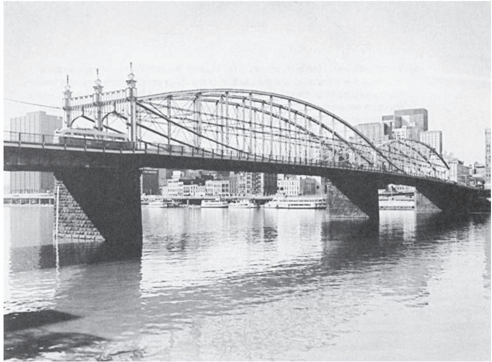
FIGURE 29 Lenticular truss: the Smithfield Stress Bridge across the Monongahela River in Pittsburgh, Pennsylvania (circa 1883).
