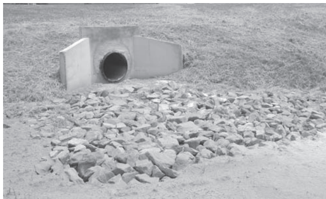
FIGURE 7.7: Culvert exit with riprap apron
